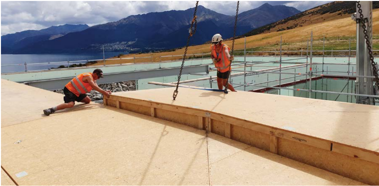
Potius Building Systems roof panel being installed
