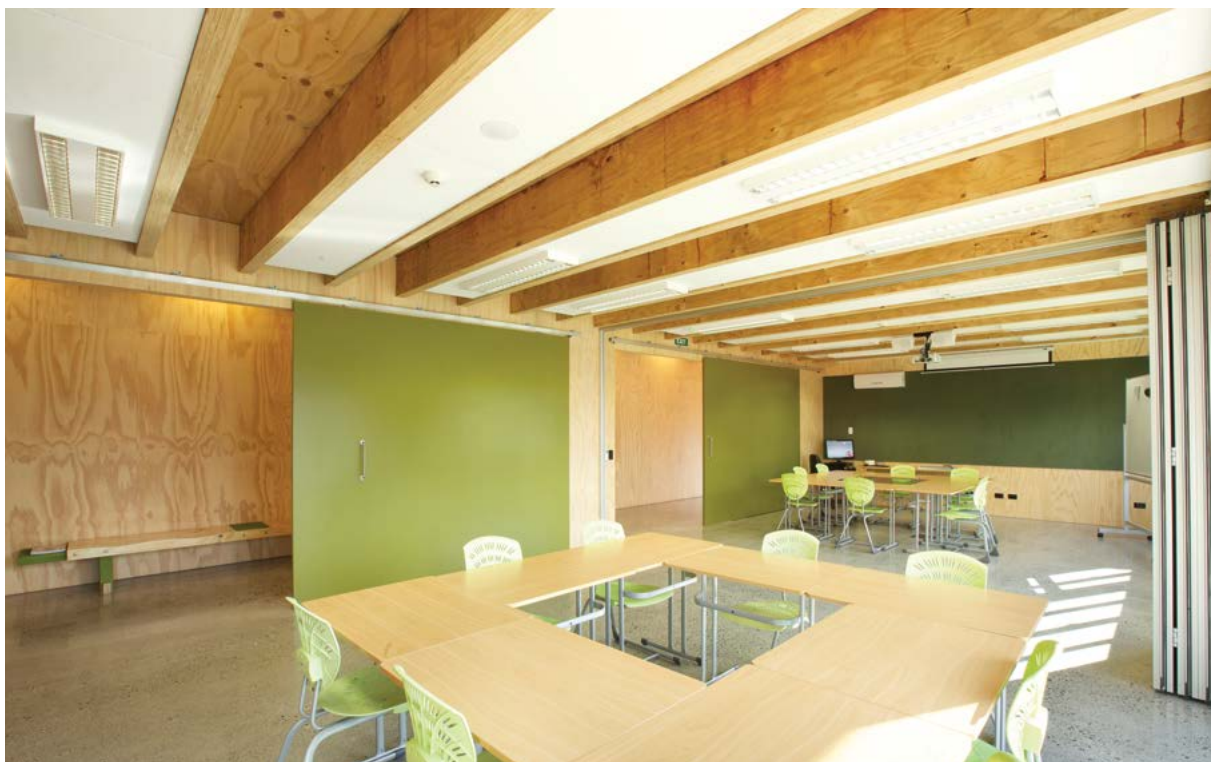
'T' panels in an educational building. In this case the webs are sized to provide fire rating.
