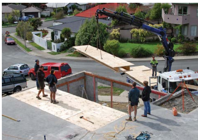
Cassettes with continuous top skins and bottom flange span full width of basement garage.
