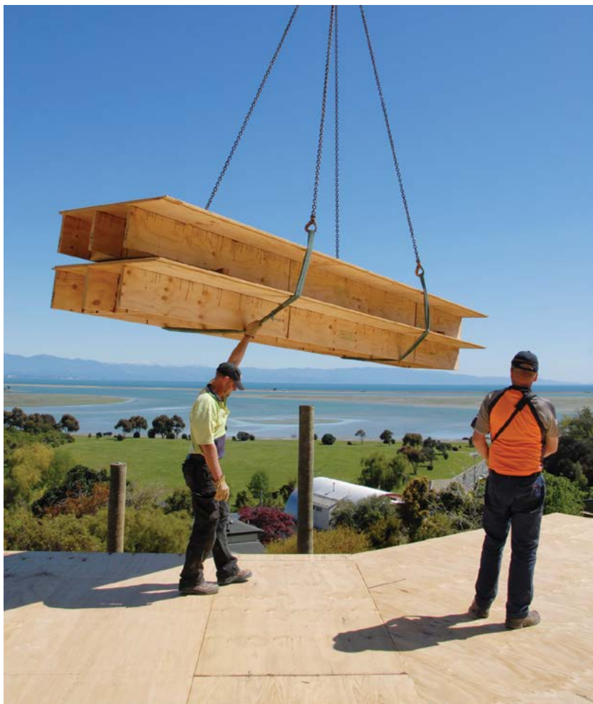
'T' panel configuration used for a residential floor in Nelson.
