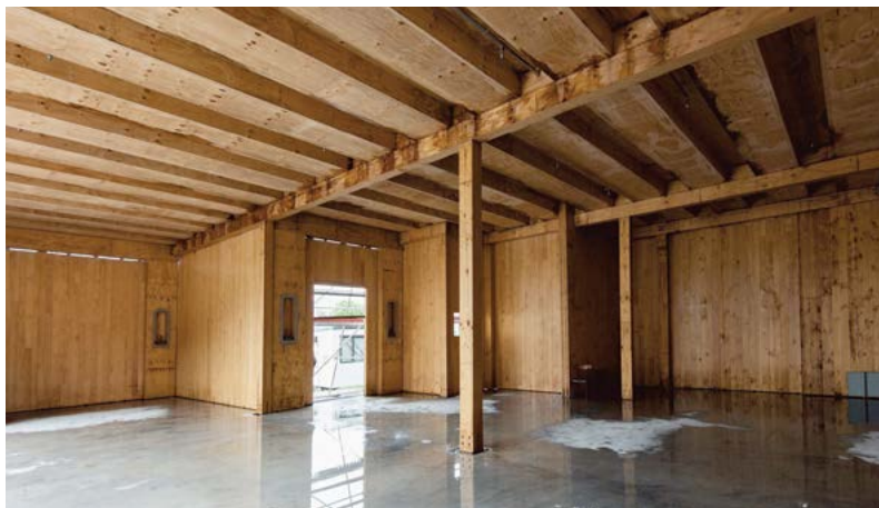
Potius box panels seated on a corbel on the face of a beam system. (Kaikoura District Council Building)
