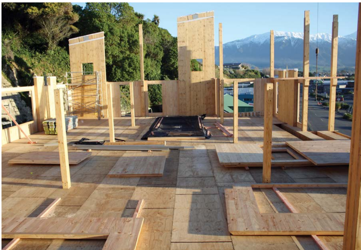
Potius floor panels in place. CLT walls layed out ready to be lifted into position. (Kaikoura District Council Building)
