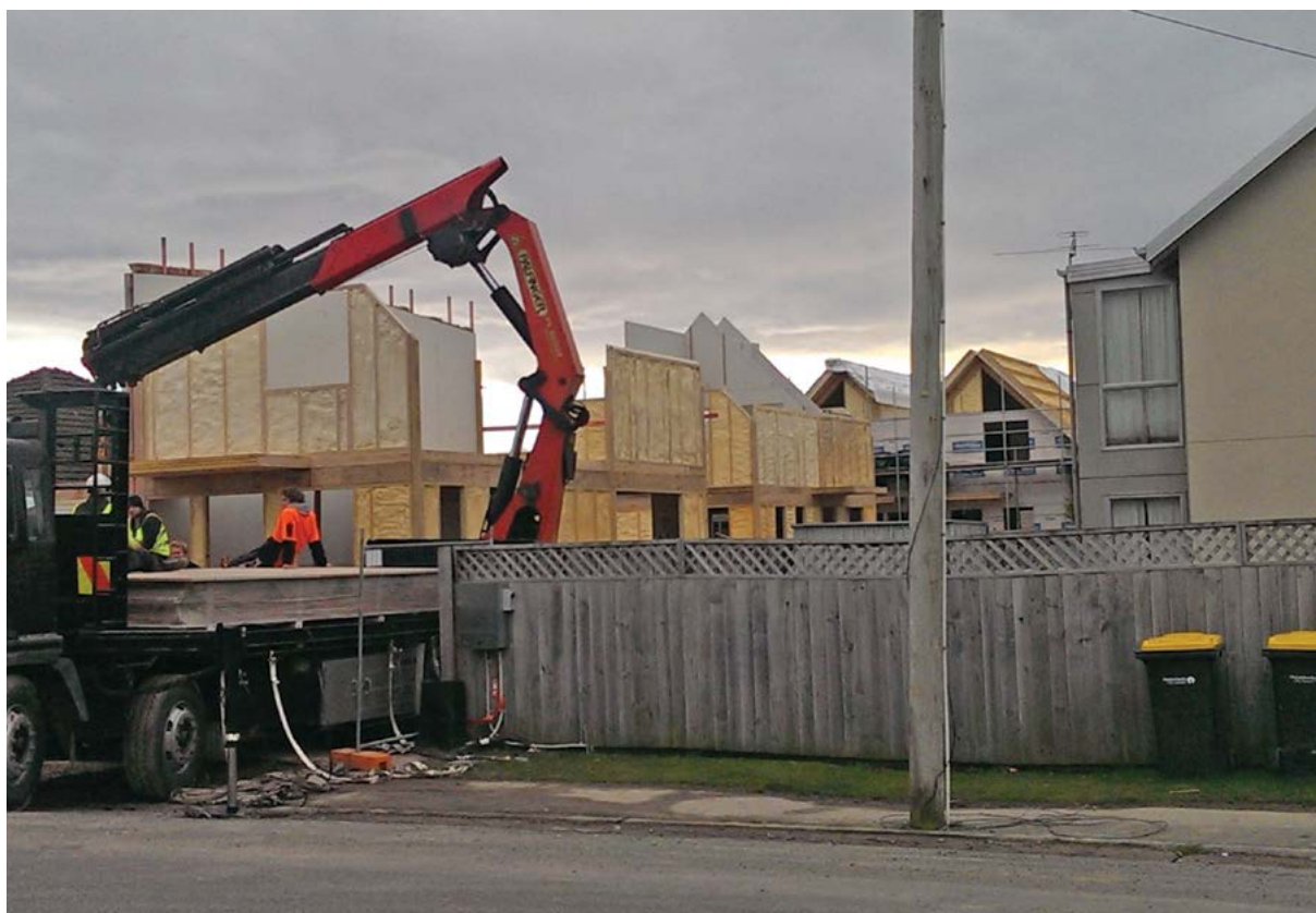
Prefabricated Potius wall cassettes with polyurethane spray foam insulation.
