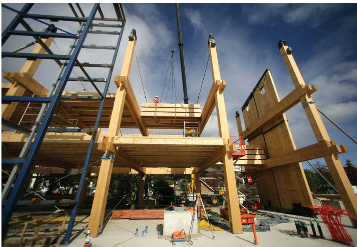
Packs of panels lifted onto beams before being unstacked and placed into final positions, minimising crane time. (NMIT Arts and Media Building)
